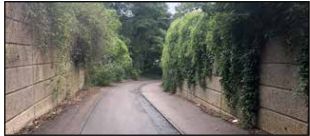
3. Looking north as bicycle path drops down through cutting
