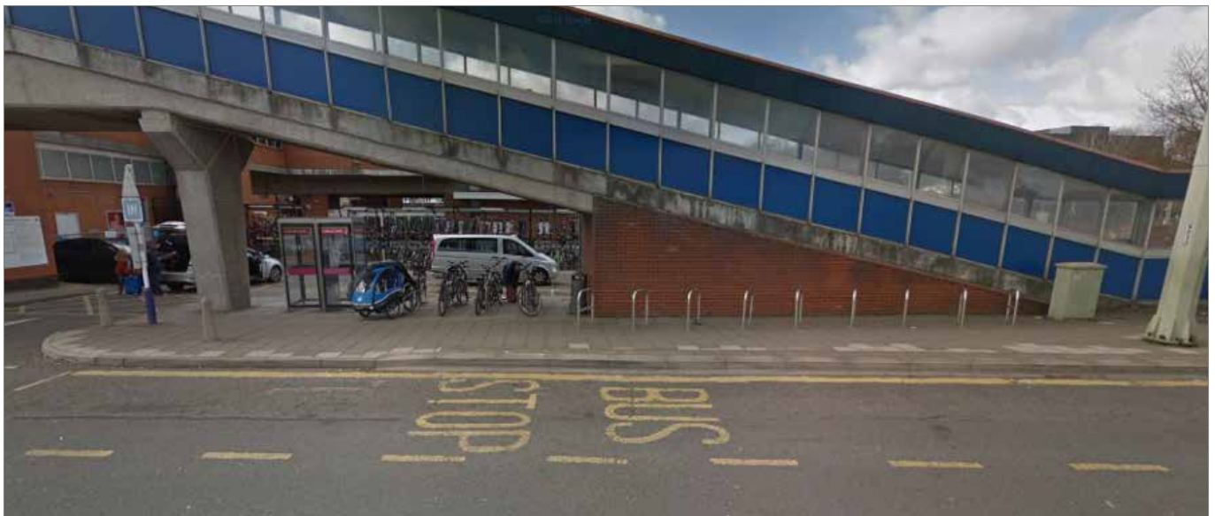
Figure 13: Walking, bike parking, bus stop and other street furniture in a small space
