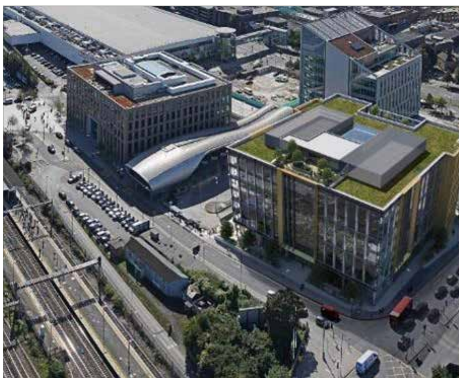
Figure 15: Station Quarter, Slough
