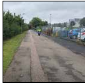
1. Looking north. Police station on right
